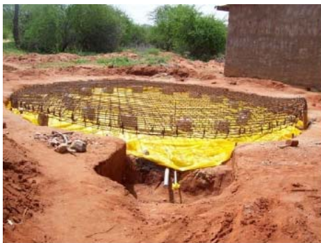
Workers are laying foundation for the first collection tank.
