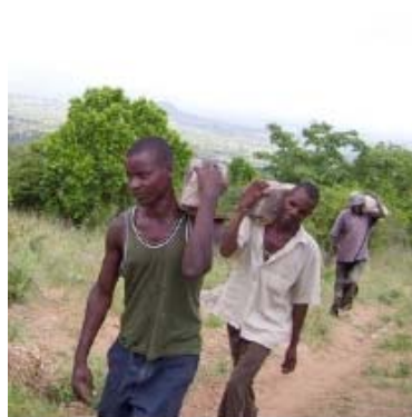
Men carry rocks for the intake chambers while women carry cement in preparation for the second collection tank. Because of the difficult terrain up on rocky hills, materials had to be ferried on the shoulders and backs of the community as no vehicle could climb up the hills to intake weir.
