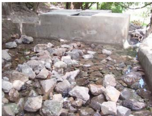
Completed intake chambers and weir.
